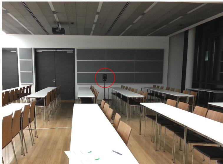
**Figure 2.4.** Lecture hall with direct sound loudspeaker in the front from a listeners' perspective. Enhancement speakers are hidden behind the grey panels in the walls and ceiling.
